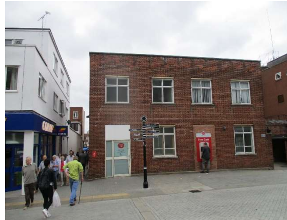
Before: back view of PO building
