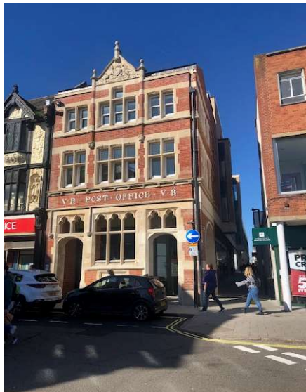
Front view of the old Post Office
