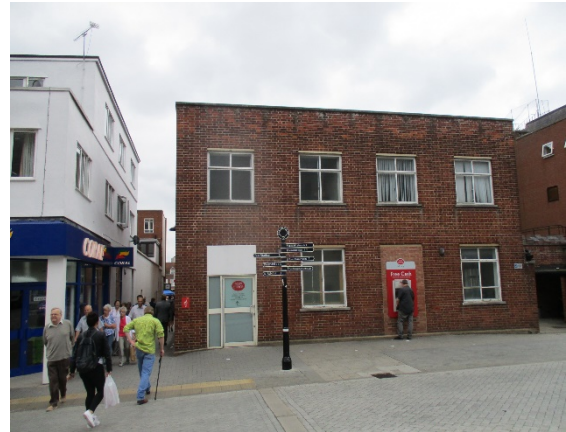
Before: back view of PO building
