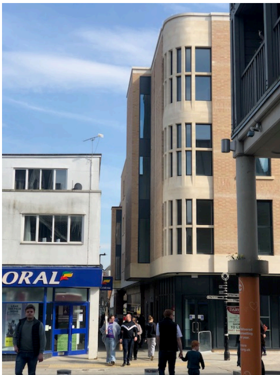
After: the rear of the building
