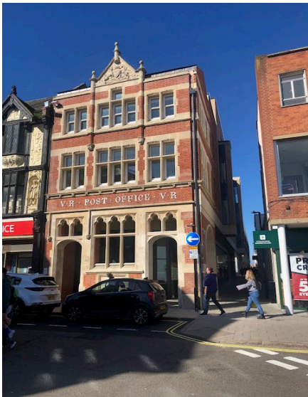
Front view of the old Post Office
