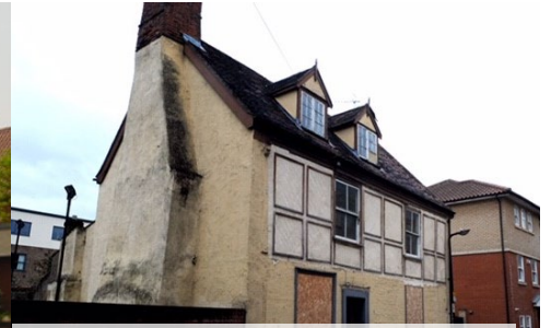
BTT's Current Project: 11 High Baxter Street
