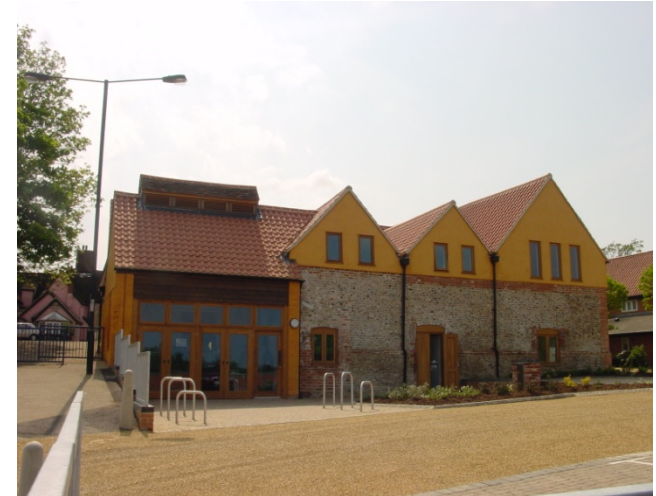
The Maltings, Bury St Edmunds Once derelict, now conserved and in full use.
