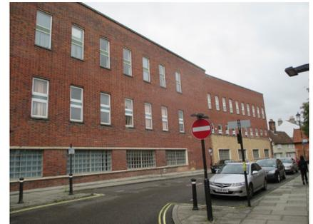
Windows are all metal framed casements with a central obscured panel. There are artificial stone copings to all brick walls and flat roofs are hidden behind parapets.
