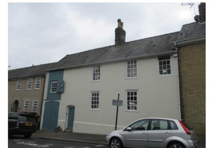
The fenestration is all with multipane sashes, which apparently are early 19<sup>th</sup> C, as presumably is the flush panelled door. Iron rainwater goods. Mounting stone (18<sup>th</sup> C?) outside at the eastern end.
